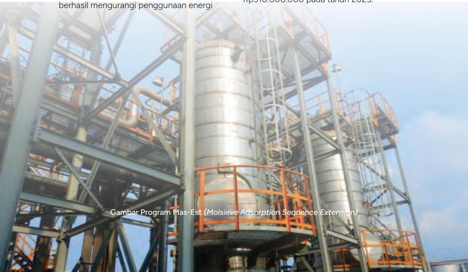
Gambar Program Mas-Est (*Molsieve Adsorption Sequence Extension*)
