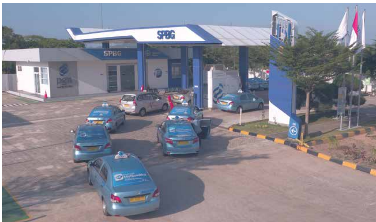
The reliability of the operation of the SPBG facility is inseparable from WIDAR's support in providing the Gas Engine Generator as an energy source for the SPBG.
