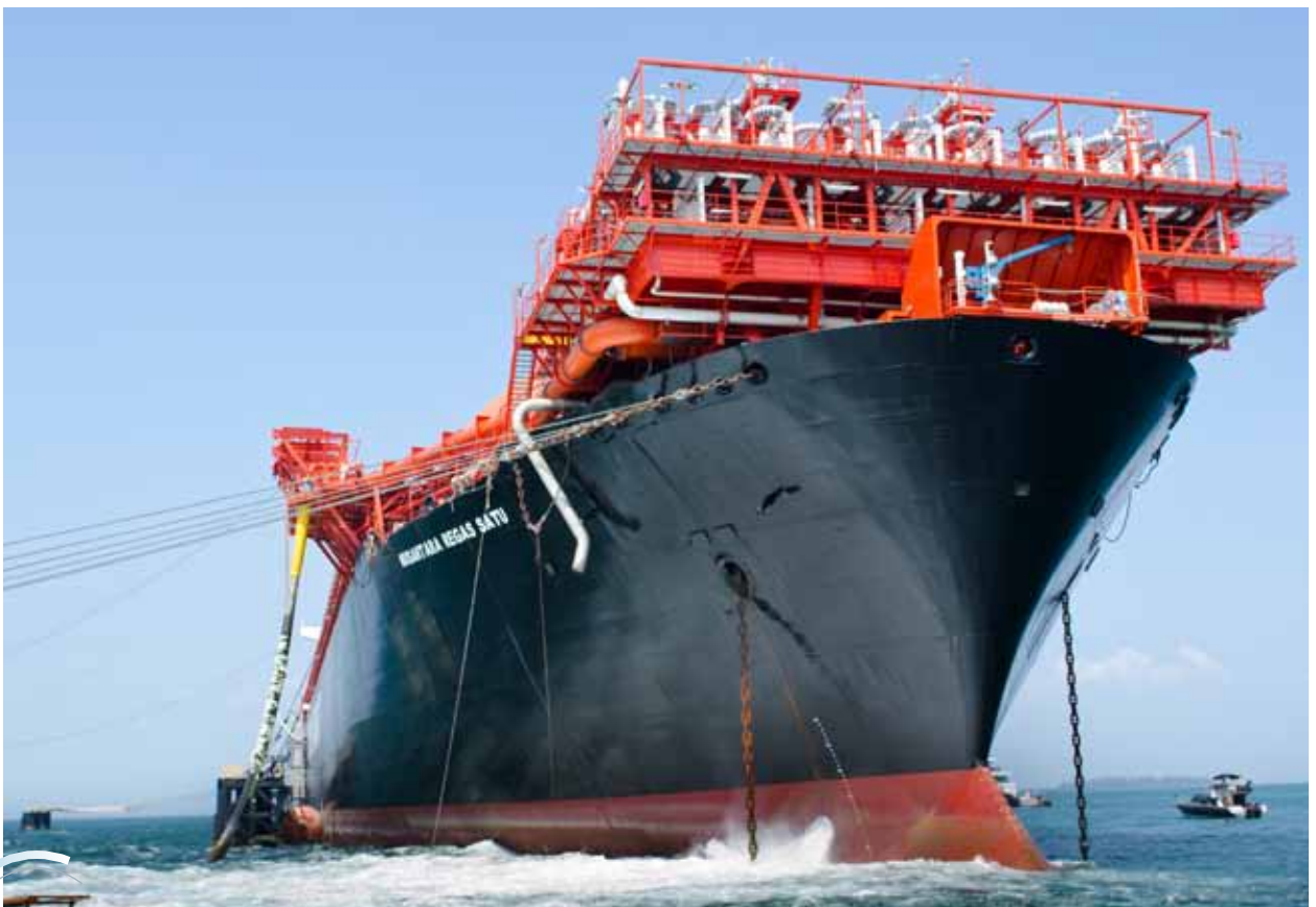
Nusantera Regas Satu, Floating Storage Regasification Unit/"FSRU" located in Teluk Jakarta has capacity of 3 MTPA
