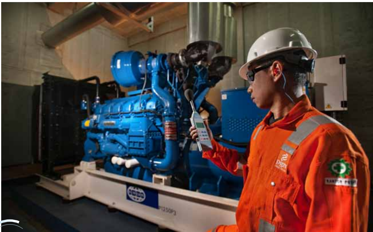
Measurement of noise level using a sound level meter at PGN's Head Office - part of the implementation of the OSH management system.
